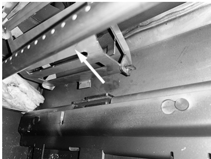
Figure 5. Remove Flue Gas Agitator
